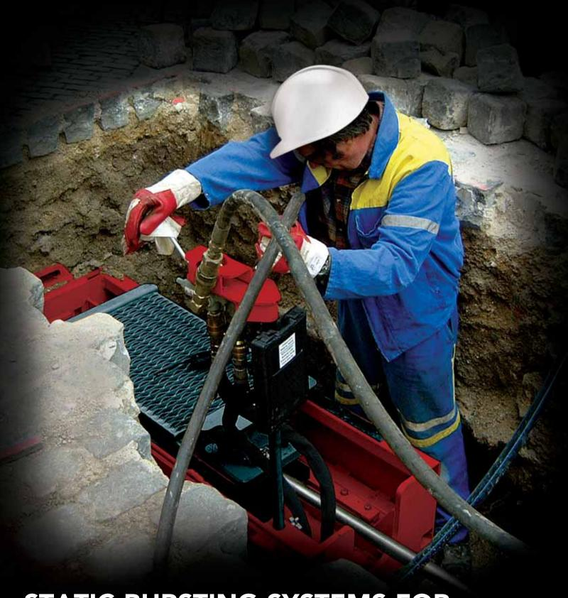
STATIC BURSTING SYSTEMS FOR GAS AND WATER REPLACEMENT.
