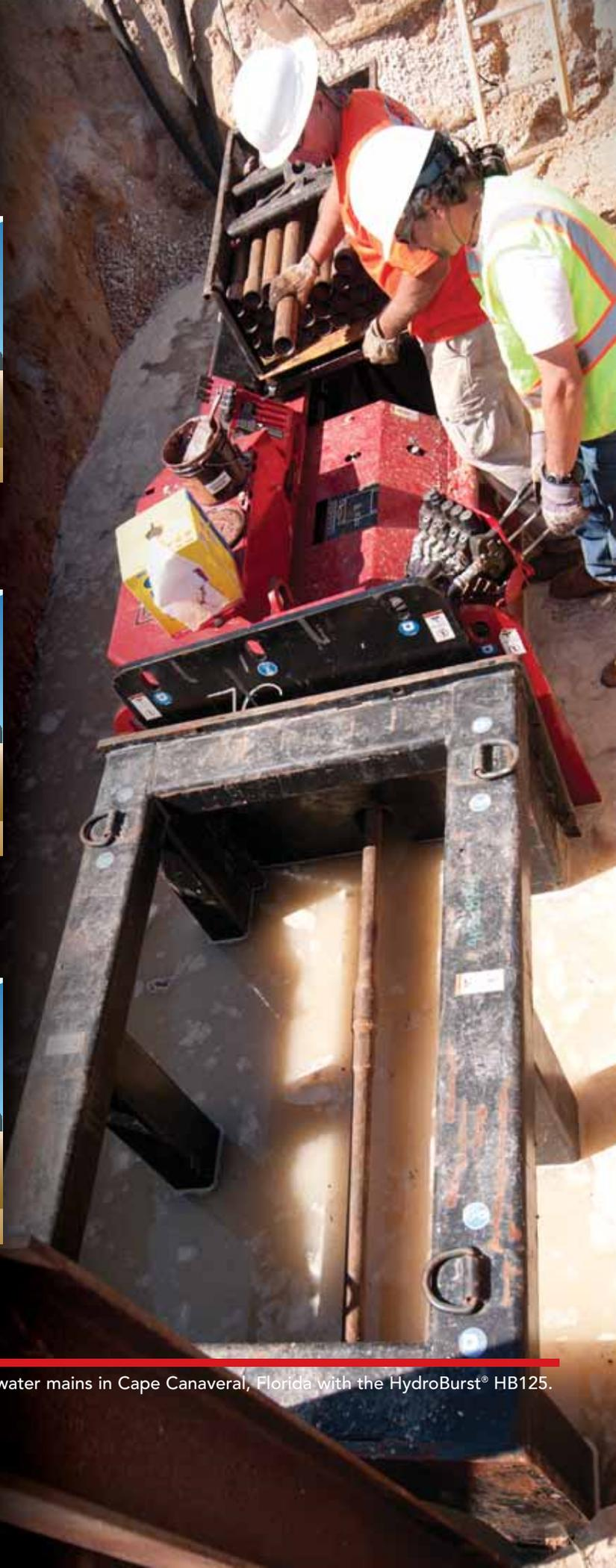
Pipe bursting water mains in Cape Canaveral, Florida with the HydroBurst® HB125.
