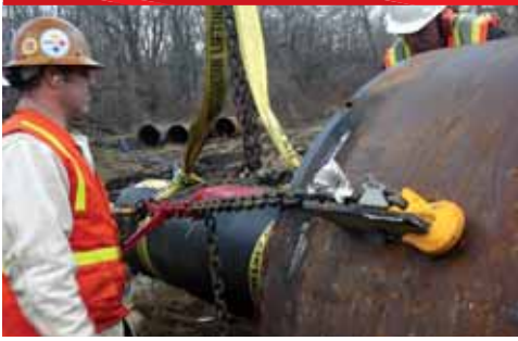
Project: New culvert under Burlington Northern Rail track Specifications: 30" & 60" steel casing Equipment: 24" pipe ramming hammer
