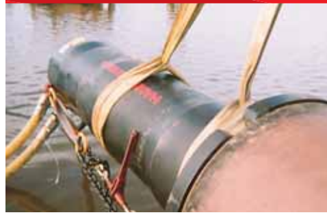
Project: Pullback assist – gas pipeline installation Specifications: 2,800' of 36" casing Equipment: 24" pipe ramming hammer
