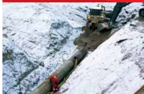
Project: Slick bore – Bannister oil pipeline project Specifications: 360' of 36" steel casing Equipment: 24" pipe ramming hammer
