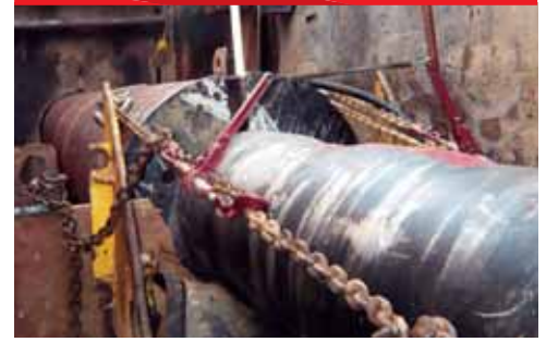
Project: Williams Gas Pipeline-West (natural gas main) Specifications: 349' of 42" casing Equipment: 24" pipe ramming hammer
