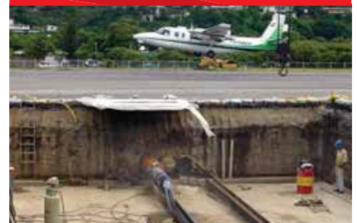
Project: Pipe bridge culvert under military runway Specifications: 26 rams of 24" steel pipe 60 meters each Equipment: 16" and 24" pipe ramming hammers
