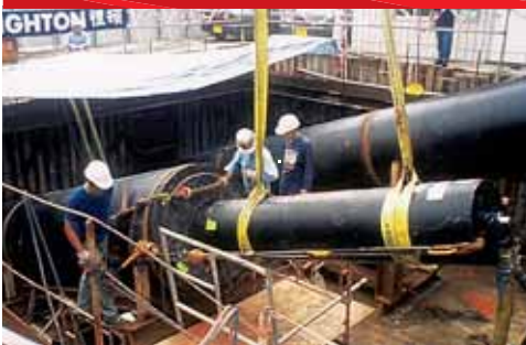
Project: Washover casing installation for HDD assist Specifications: 2 – 54" casings 66' at a 20° angle Equipment: 24" pipe ramming hammer
